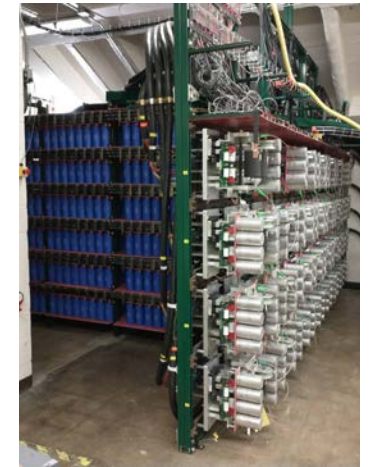
New TF/PF Energy Storage and Switchyard Built
