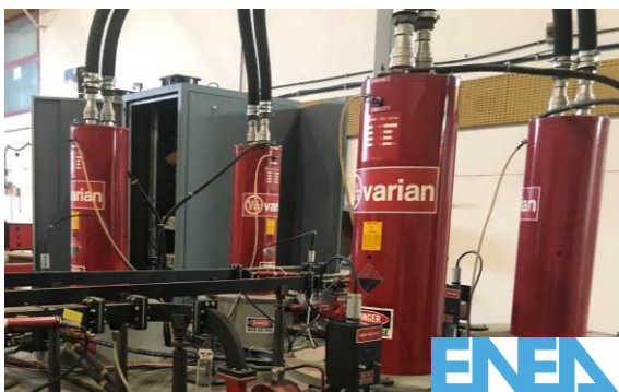
Klystrons powered by new DC-DC resonant supplies
